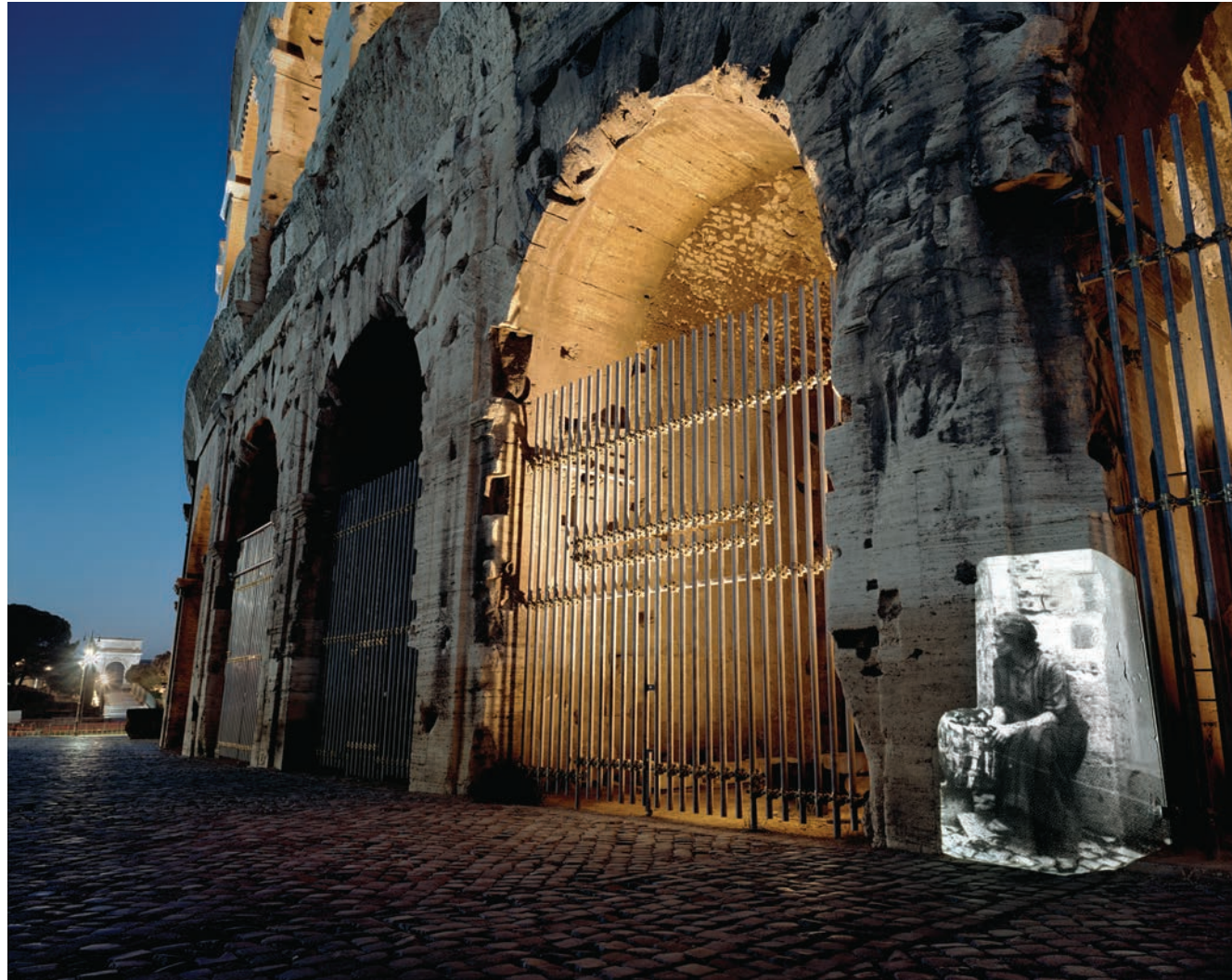
At the Coliseum (Looking towards the Arch of Titus) from The History of Another, 2003
