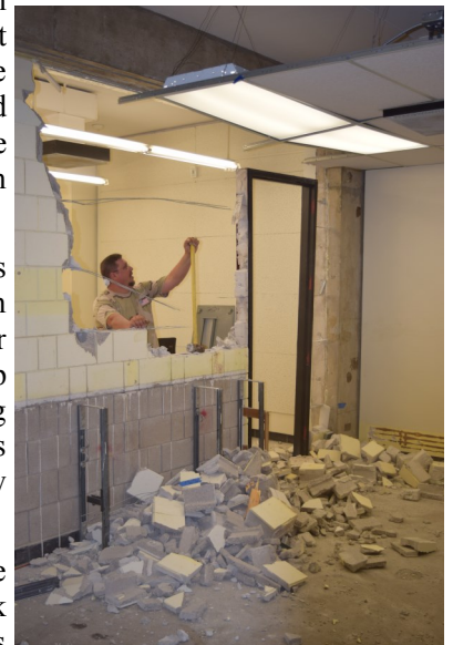
Demolition began in September.
