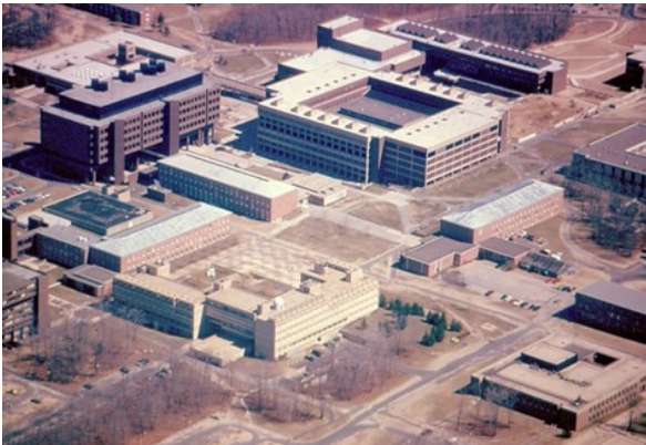
Aerial view of the brand-new ESS Building, 1968
