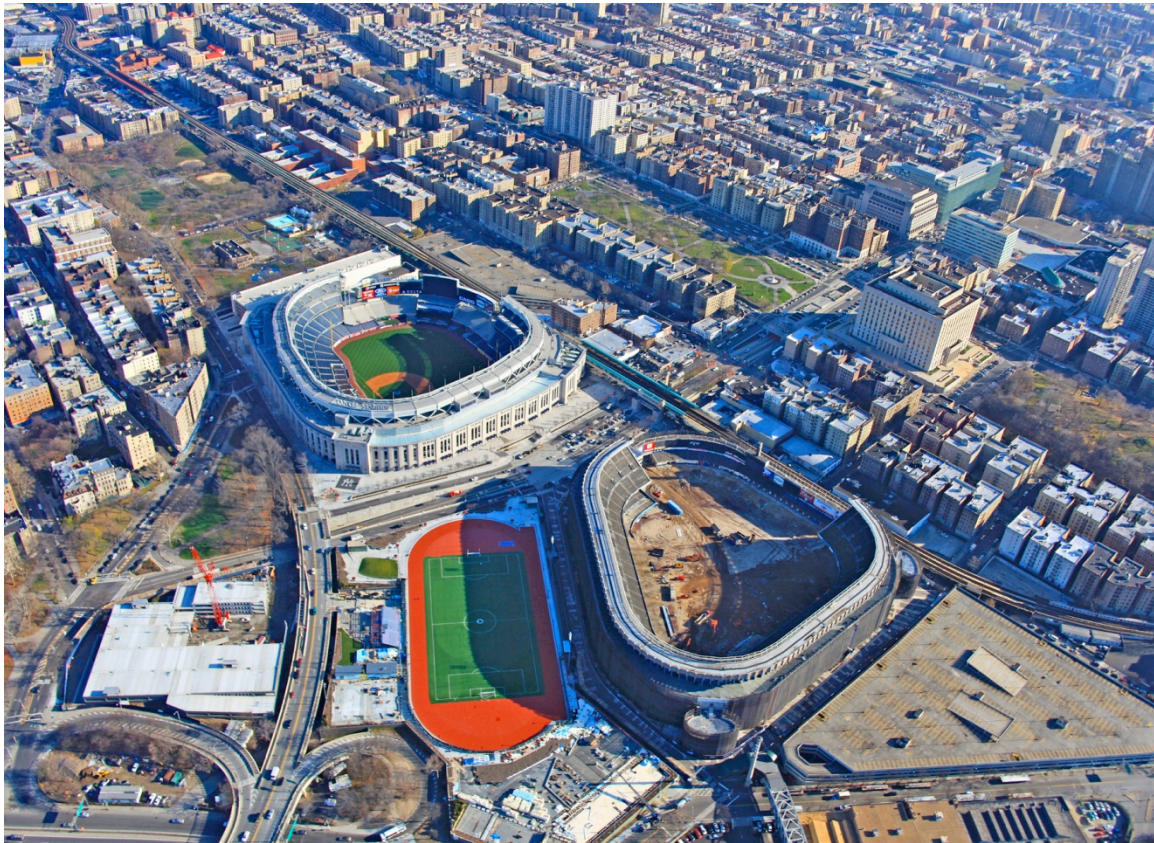
Figure 1 – New Yankee Stadium built to the north of the old stadium. Photo taken in 2010 shows the old stadium starting to be demolished. Rock outcrops are present under the trees at the center right and center left edges of the photo. (Digital image from MRCE archives.)
