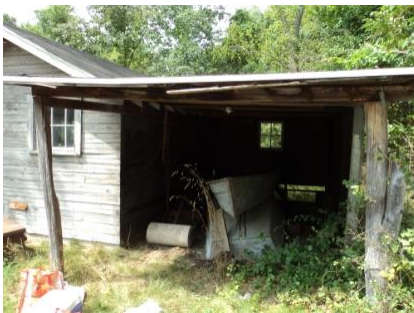
Figure 12: 100+ year old Boathouse where undisturbed soil samples were collected.
